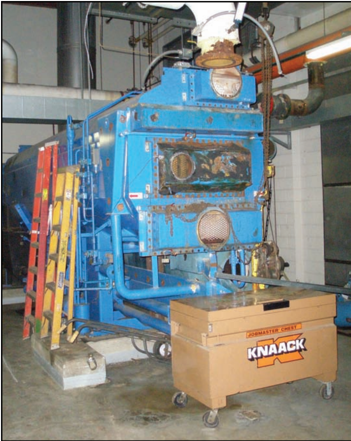
FIGURE 5. The last of the old chiller-heater before demolition.
